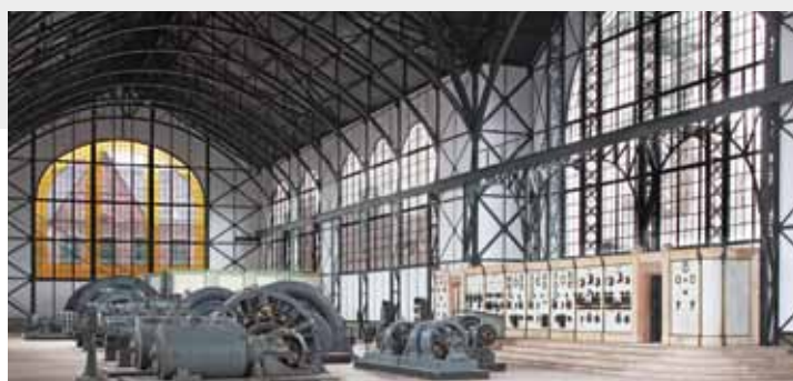
Inside view of the engine house
