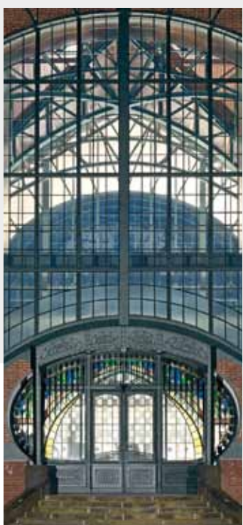
Entrance of the engine house
