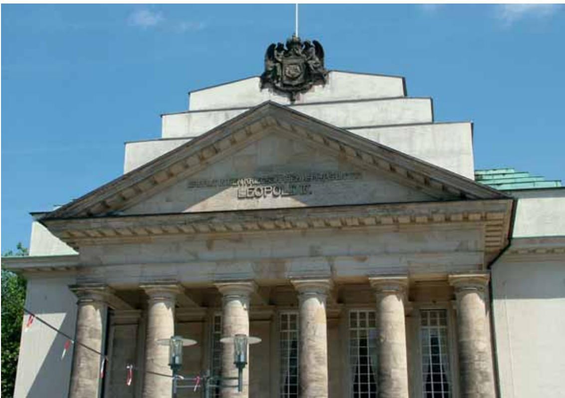
Abb. 32: Landestheater in Detmold (1914 – 1916)
